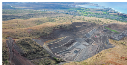
[Landfill Application, Hawaii]
