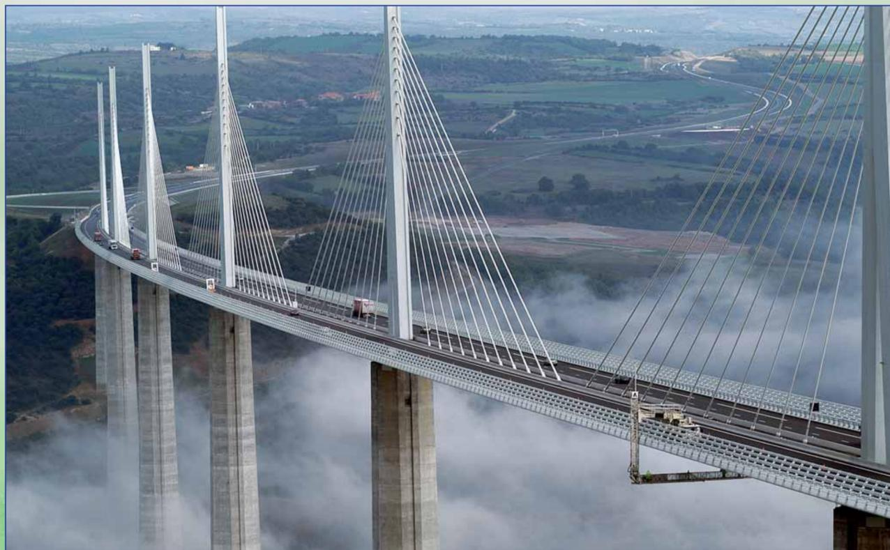
The products of the "ABC line" for inspection and maintenance of road bridges guarantee a safe, quick and economic system of access to those structures where setting up of scaffolds is not feasible or it is too costly. The ABC units, mounted on standard trucks or trailers, take a few minutes only to deploy from the rest position to the work position, without personnel on board.
