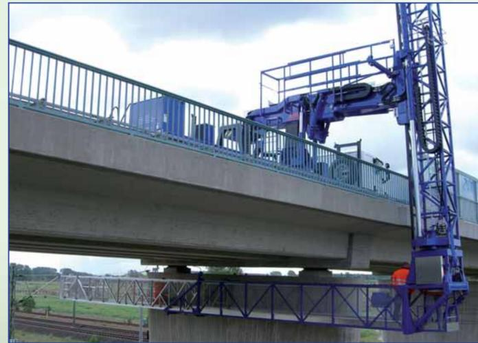
The spacious platforms of the ABC range of machines enable the operators to carry out any sort of heavy-duty repair work underneath bridge decks, by the use of electric/hydraulic/pneumatic operated tools which can be supplied directly from the outlets provided on board the platform. Demolition works can be carried out as well by means of hammers, by previous protection of the platform with plastic covers against the fall of debris.
